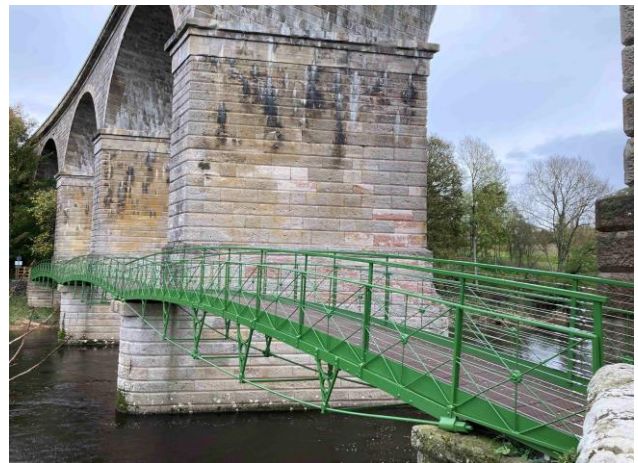
Image: Roxburgh Viaduct Footbridge
