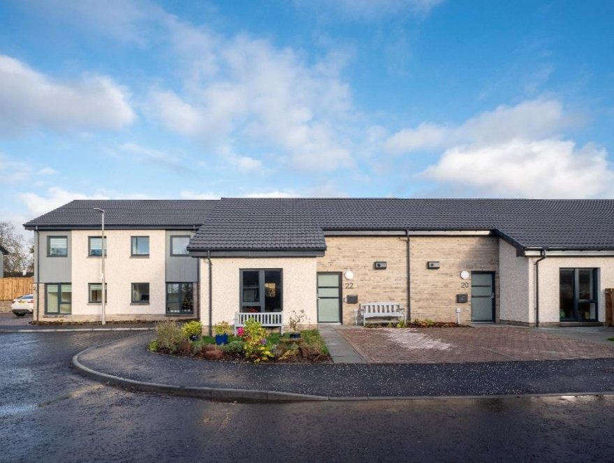
Figure 4 Photograph of completed Passivhaus Development © McAteer Photo & ECD architects
