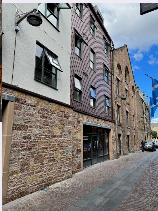
Rear of building, Baron Taylors Street - before and after
