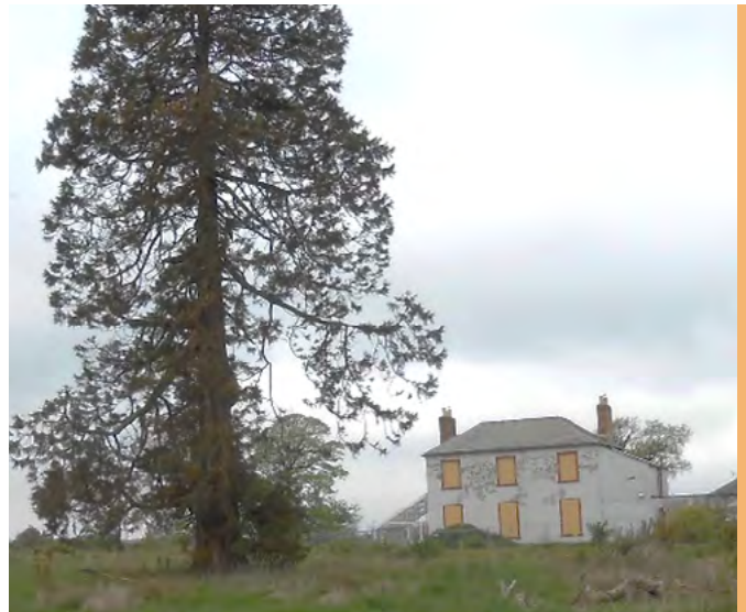
Longmeadow House before restoration
