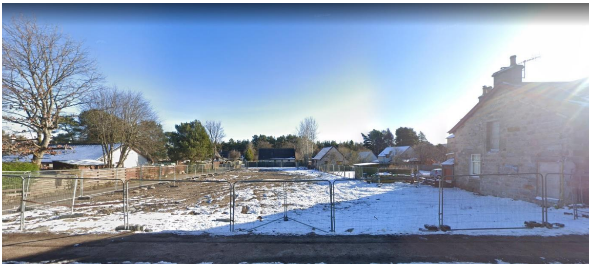
The site following the demolition of the Struan Hotel, March 2023 © Google Street View.
